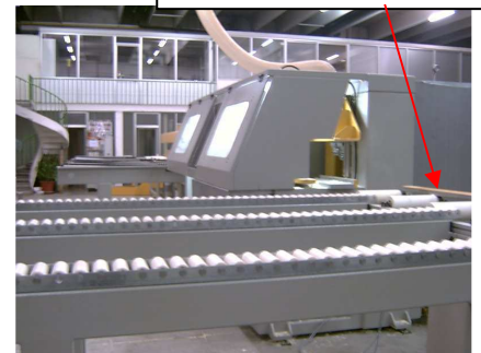
Outfeeding basement with motorised rollers
