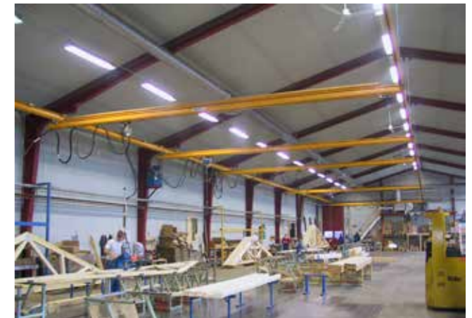
Press line in light overhead crane
