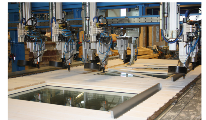
The nail pushers are desynchronized by a fraction of a second in order to not damage the frame work and to still maintain a high capacity.
