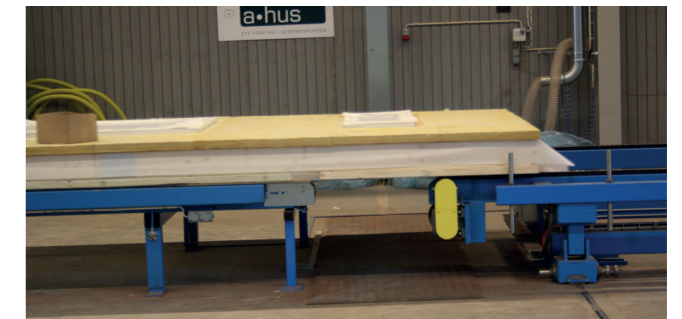
Safety mats between the stations eliminates the operators to get pinched between the station and a moving wall element.
