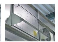
6 Explosion-flaps with flame deflectors allow an immediate pressure release. The highest degree of safety is ensured by additional safety position switches for continuously monitoring the system and shutting off the plant in case of an emergency.
