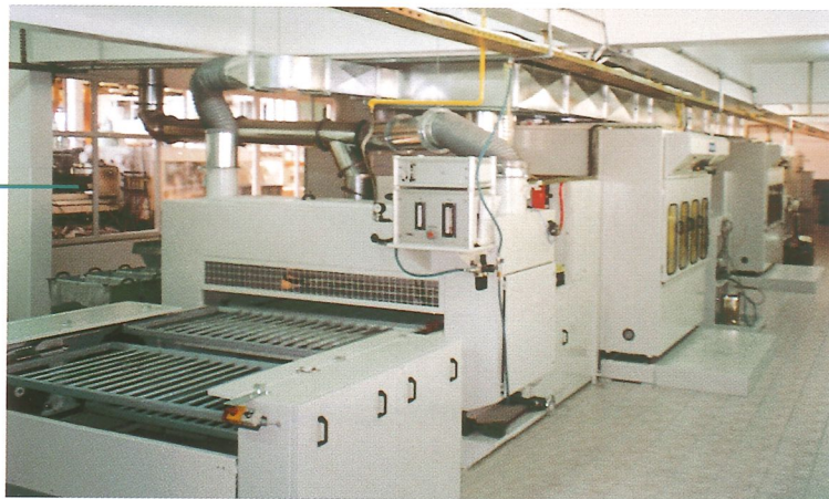
Finishing installation with pallet conveyor system and drying for plastic parts
